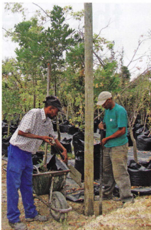
Employees Michael Fortuin and Victor Kuiken hard at work in the nursery cementing down a pole that will accommodate an overhead sprinkler.
